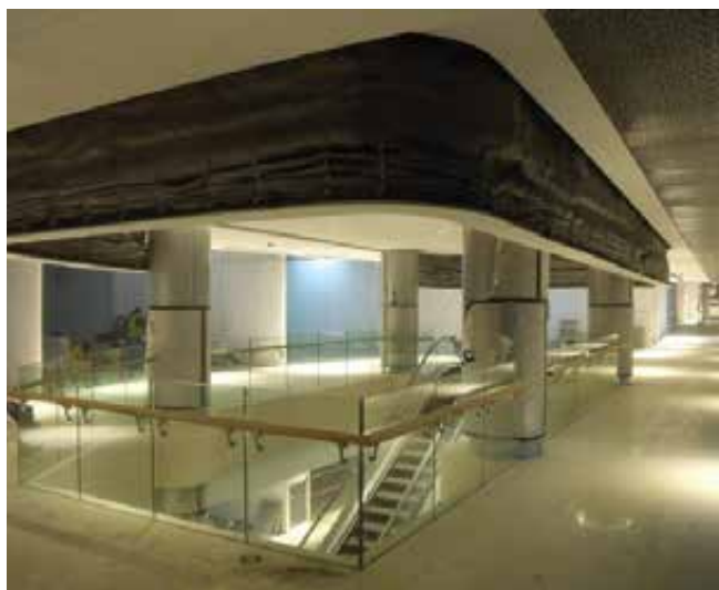
Fire rated fabric shutter at ION Orchard. In the event of a fire, these shutters confine the flames and prevent spreading.
